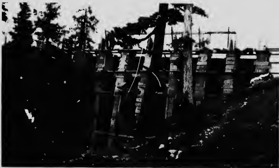
Britannia Mining and Smelting Company, Limited. Downstream face of Utopia Dam during construction.
